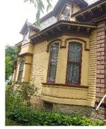
Brown's Mansard-roofed cottage posed a stylistic problem. It was essentially a story and a half structure. The steep roof covered most of the second floor, allowing for ten-foot ceilings. However, windows in the roof area were traditionally set above the cornice, creating a claustrophobic interior.
